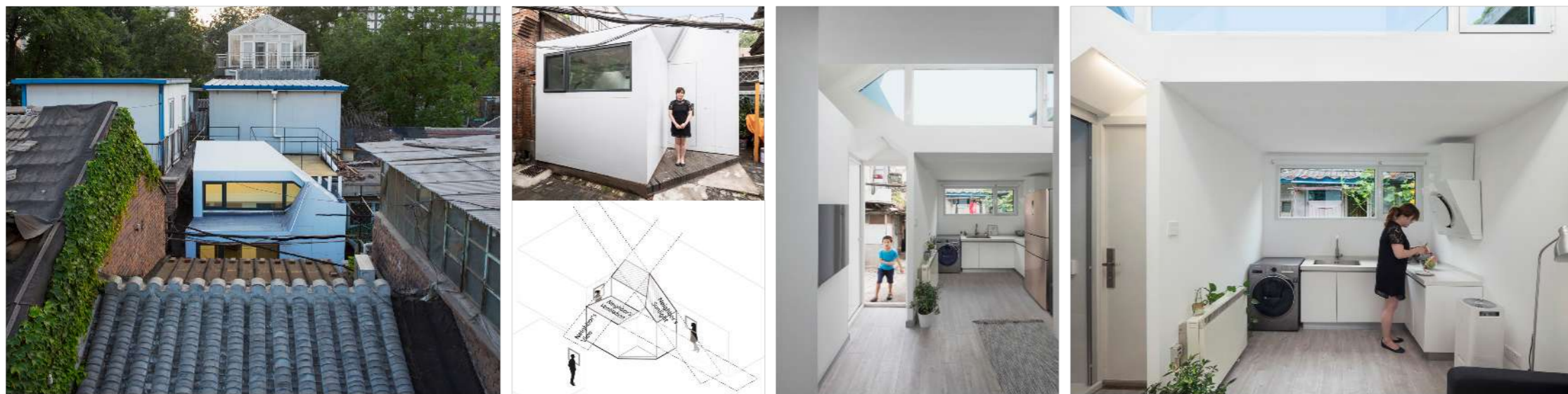
Mrs. Fan's Plugin House: the exterior form is determined by neighbors' requirements for sunlight and ventilation while the interior is light-filled and airy.
